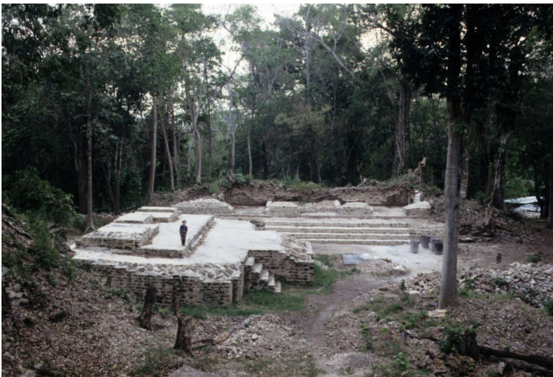
Figure 7. Caracol Central Acropolis stabilization undertaken by the USAID efforts (looking south).
