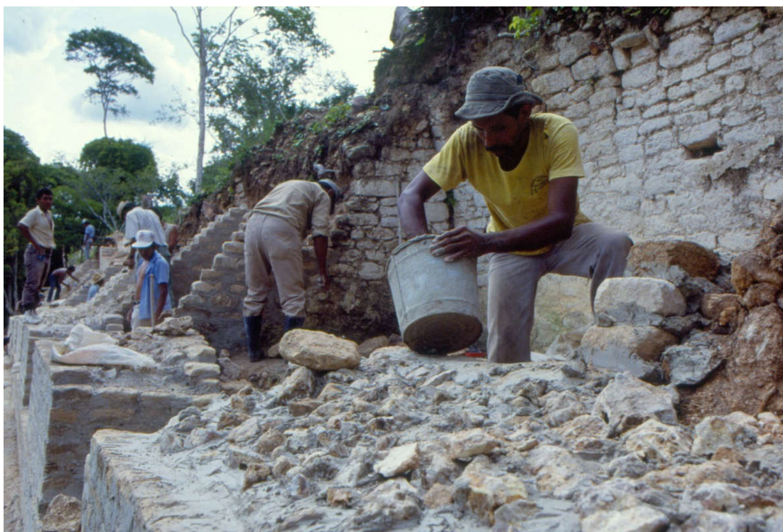
Figure 8. Stabilization being undertaken on the front face of Caana by the USAID efforts.
