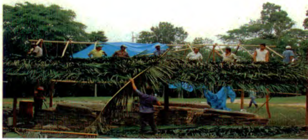
Workmen construct the thatch roof of a temporary structure that protects the monuments found at Caracol.
