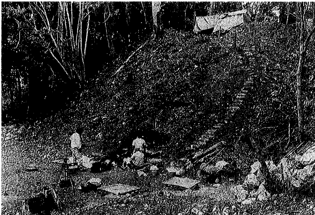
Figure 3. Initial investigations into Structure A34 showing the test excavation at the base of the substructure in which the lower tomb was found.
